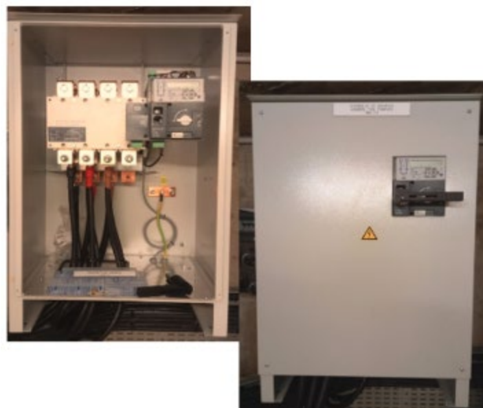
Raccordement des coffrets
