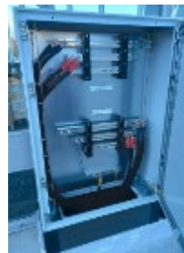
Raccordement des coffrets
